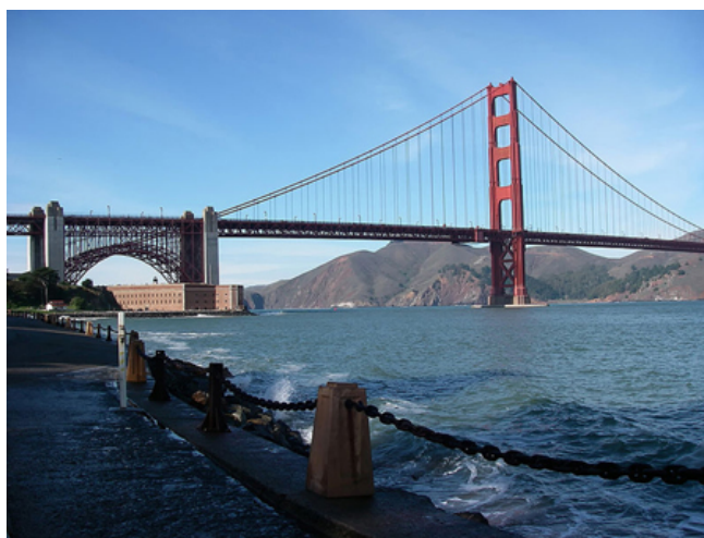
Figure 4.20 Unless an infinite tension is exerted, any flexible connector—such as the chain at the bottom of the picture—will sag under its own weight, giving a characteristic curve when the weight is evenly distributed along the length. Suspension bridges—such as the Golden Gate Bridge shown in this image—are essentially very heavy flexible connectors. The weight of the bridge is evenly distributed along the length of flexible connectors, usually cables, which take on the characteristic shape. (credit: Leaflet, Wikimedia Commons)
