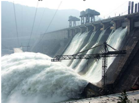
Figure 7.38 Hydroelectric facility (credit: Denis Belevich, Wikimedia Commons)
